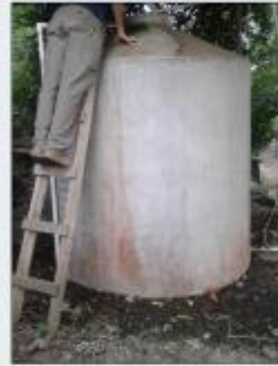
Wood Processing Plant Tank
