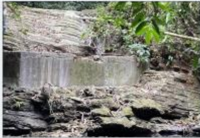
Former Collection Structure
