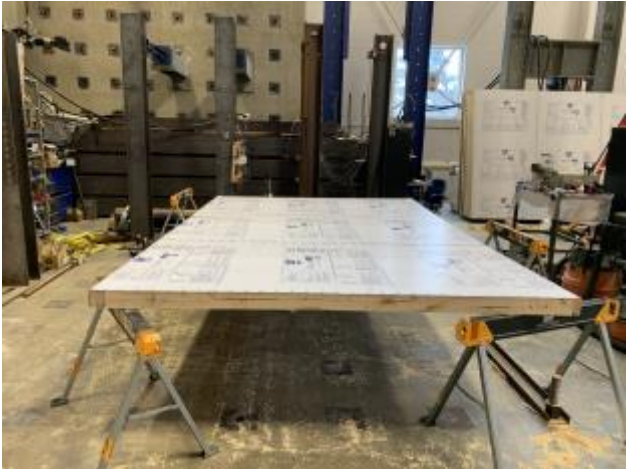
2 - Setup of wall to drill holes for testing connection
