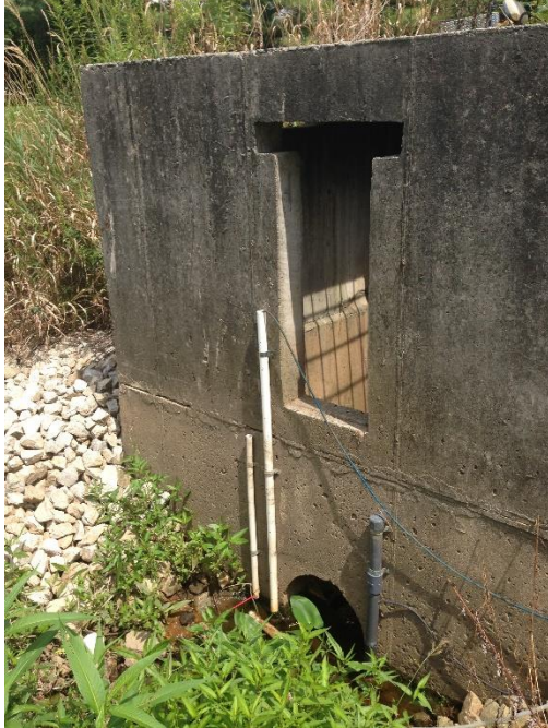
Figure 15: Outlet structure of the stormwater wetland
