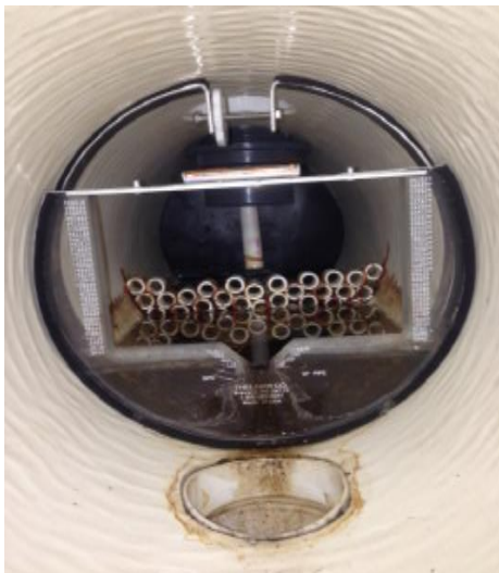
Figure 2: Interior of the green roof overflow weir box
