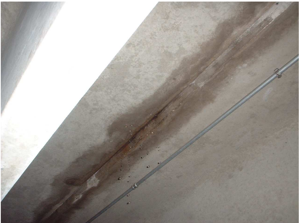
Figure 4-2: Leaking parking deck joint.
