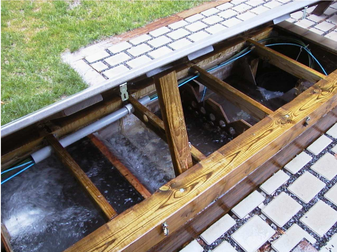
Figure 1-6: Pre-treatment sedimentation box at the infiltration trench.
