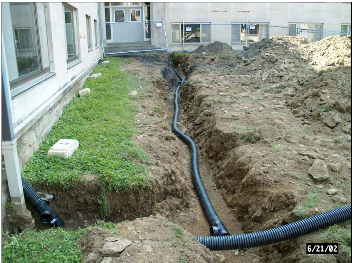
Figure 14. HDPE pipes connecting downspouts
