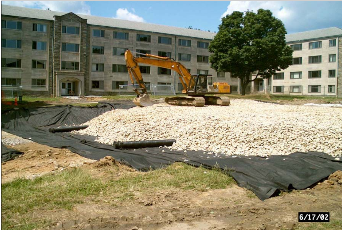
Figure 8. Middle infiltration bed under construction
