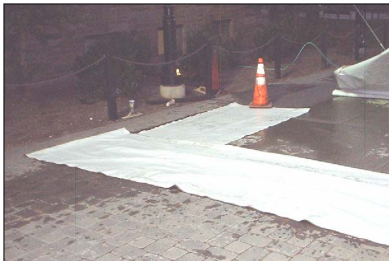
Figure 21. Wet burlap covering porous concrete
