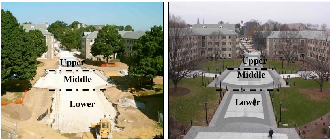
Figure 6. Infiltration bed locations during and after construction
