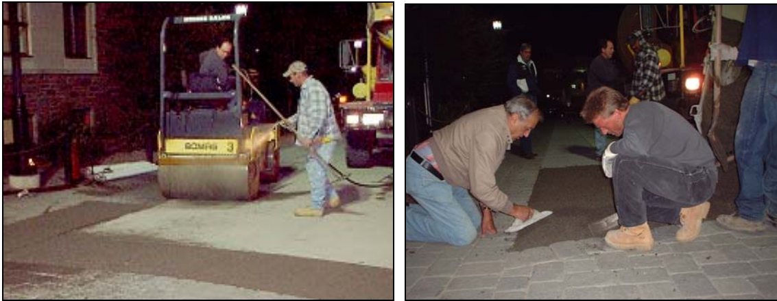
Figure 20. Rolling (left) and hand trowelling (right) of new porous concrete
