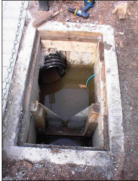
Figure 11. Weir outlet control structure
