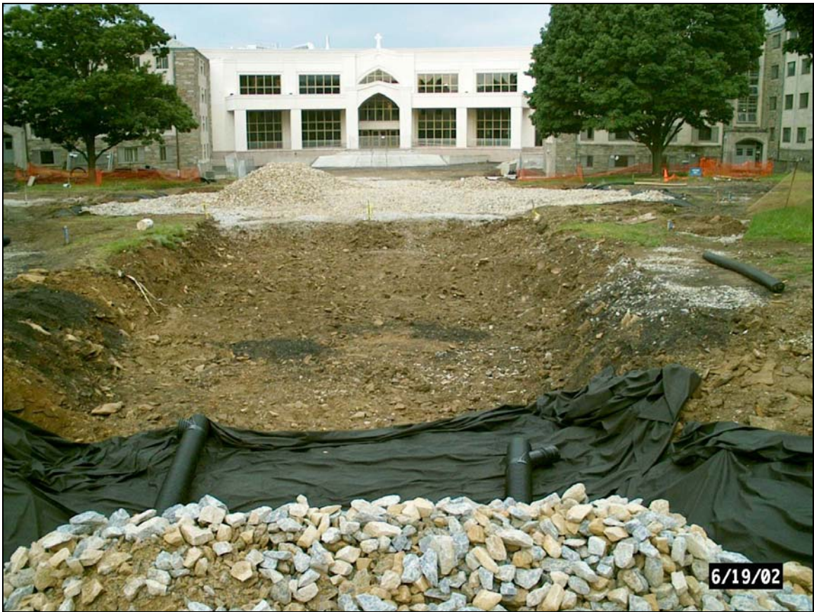
Figure 13. Upper infiltration bed mid-way through construction
