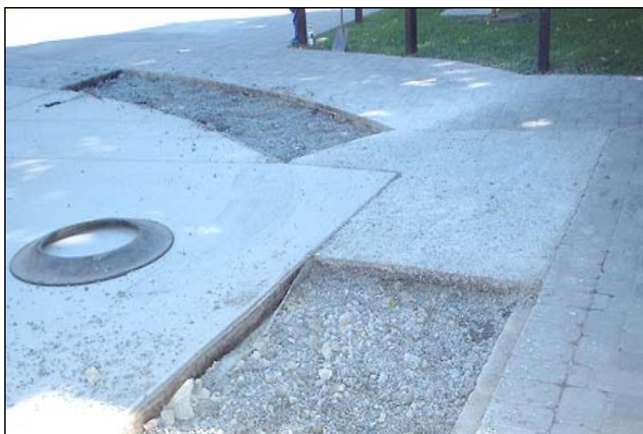
Figure 19. Sections of removed porous concrete
