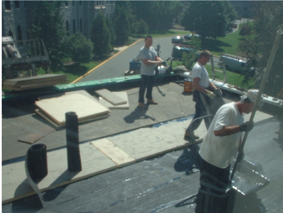
Figure 16. Installation of insulation and impermeable membrane
