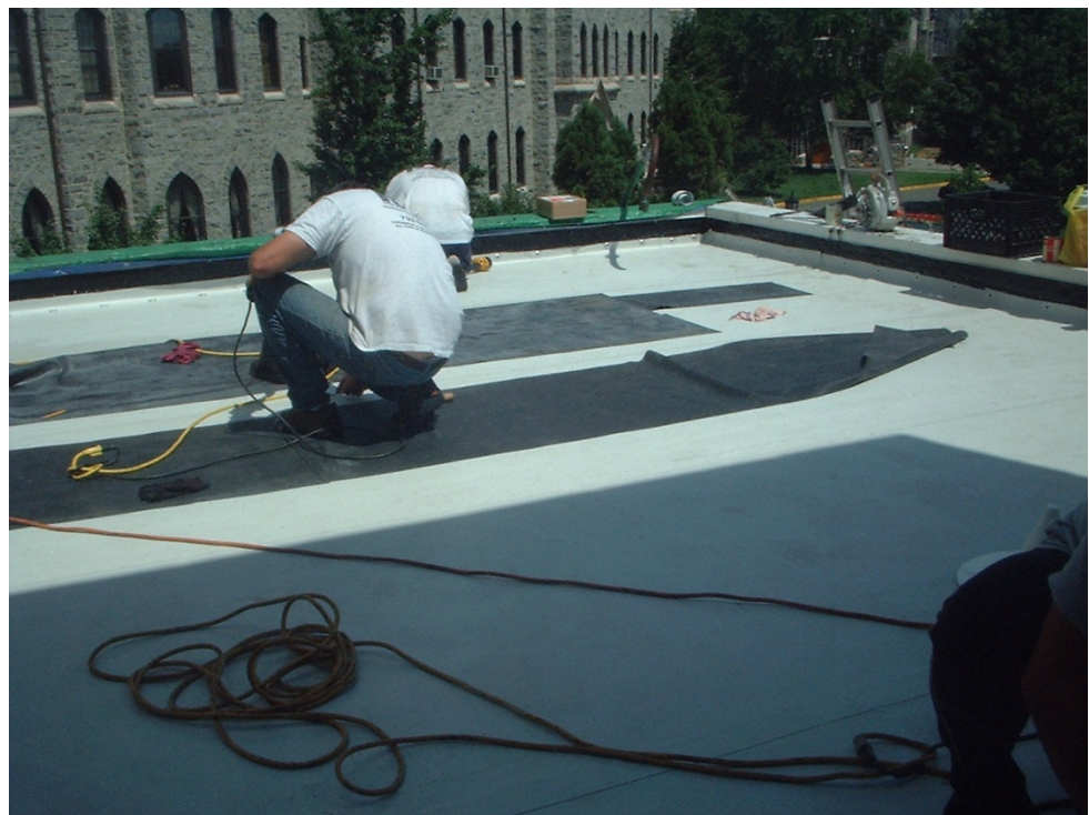
Figure 15. Installation of building protection matting
