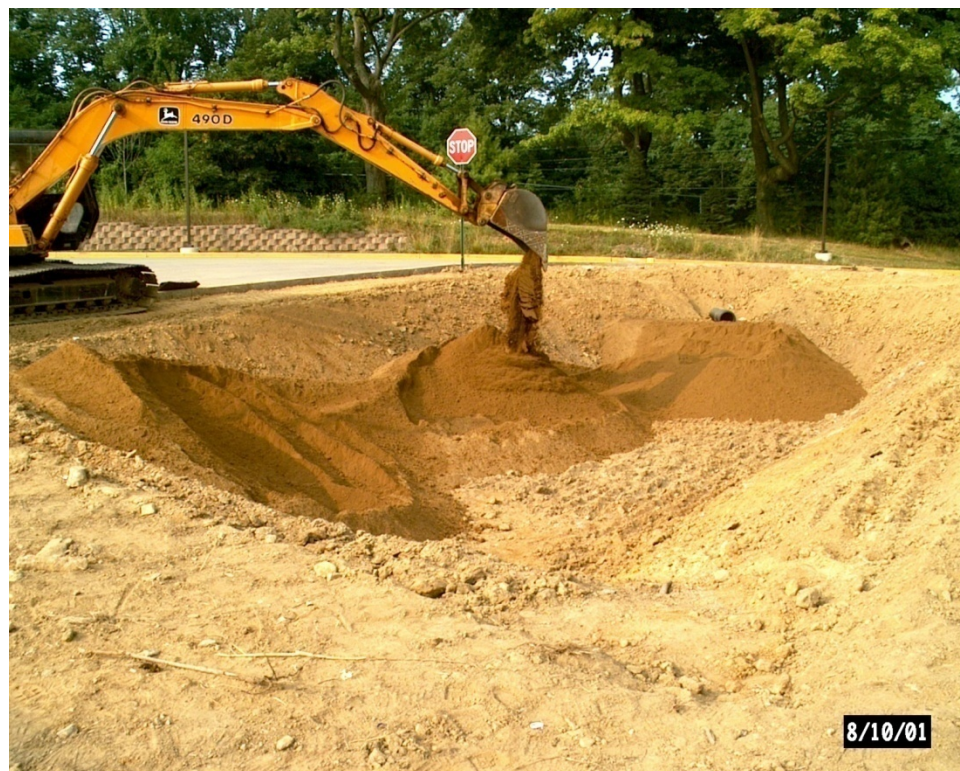
Figure 7. Excavated area backfilled with four feet of rain garden media
