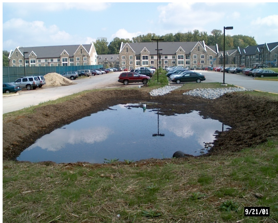
Figure 9. After application of shredded hardwood mulch as surface cover
