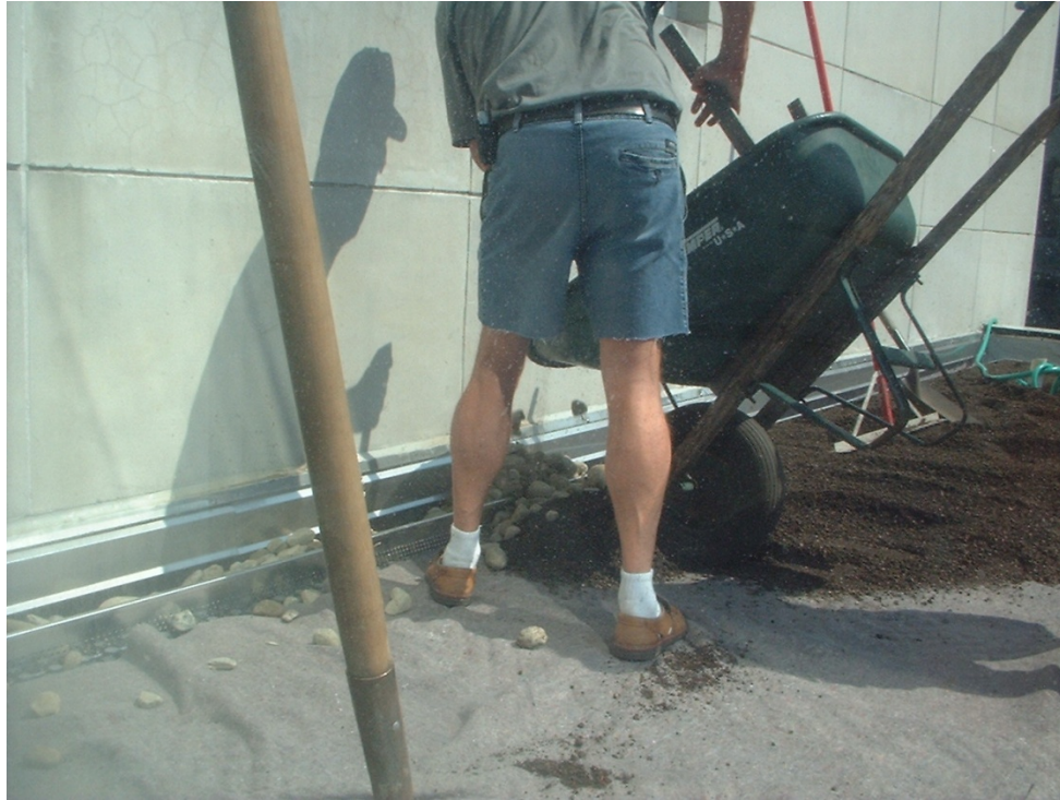
Figure 20. Addition of stone to green roof edge drain
