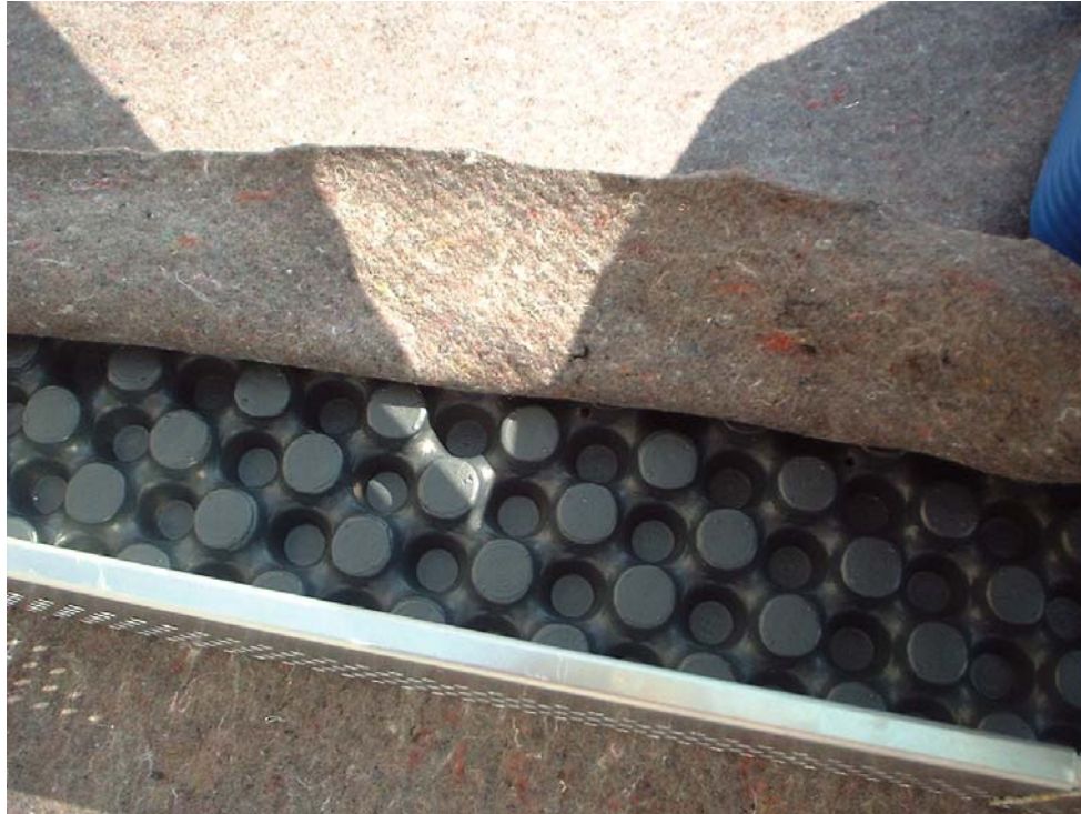
Figure 18. Installation of drainage and filter fabric layers
