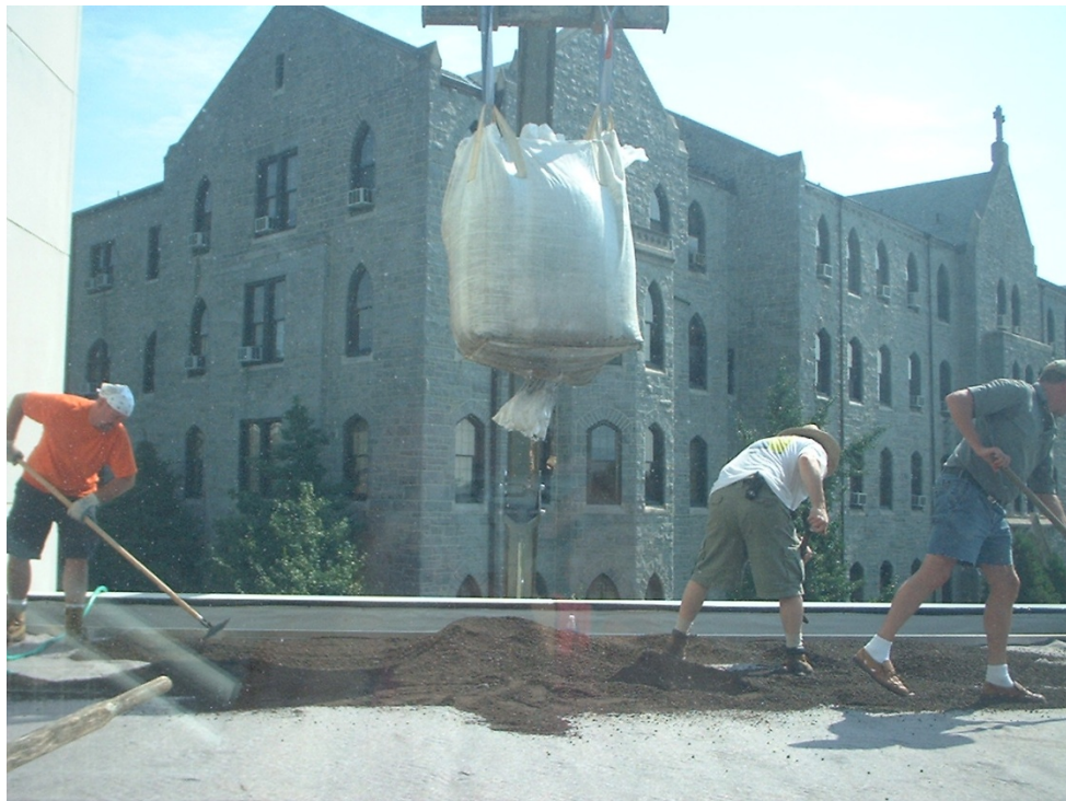
Figure 19. Application of green roof media
