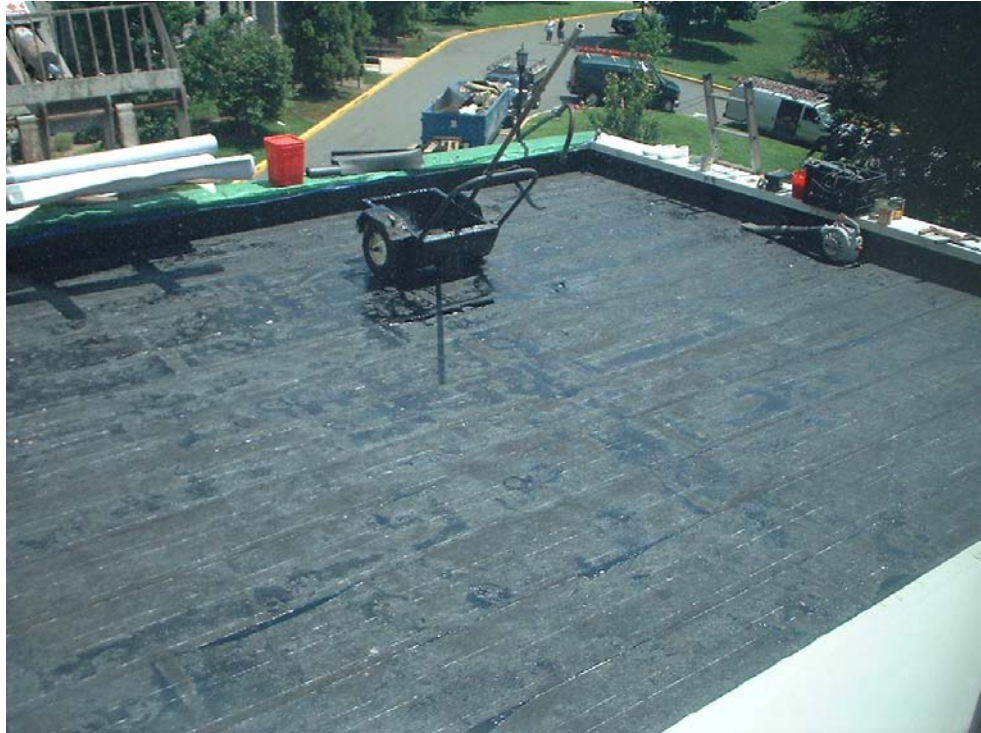
Figure 14. Resealing of existing roof
