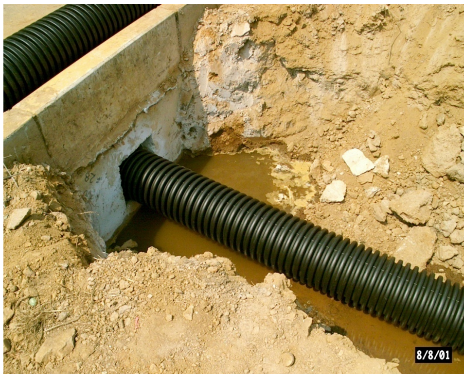
Figure 5. Roadway inlet diversion installation
