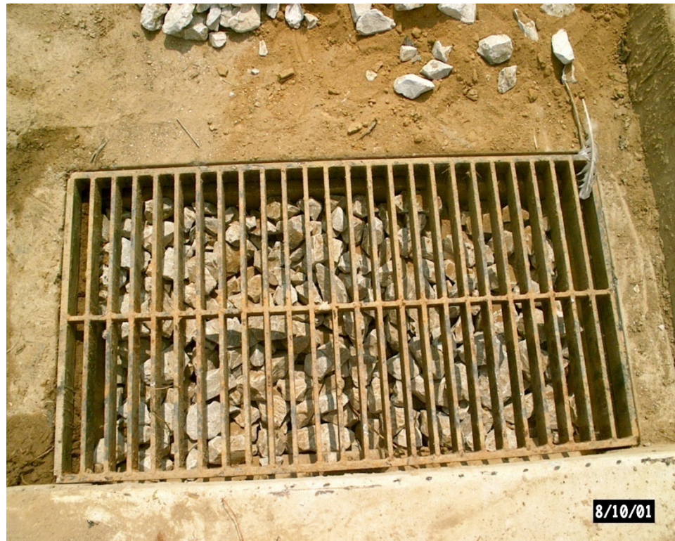
Figure 8. Filling of existing parking lot inlet
