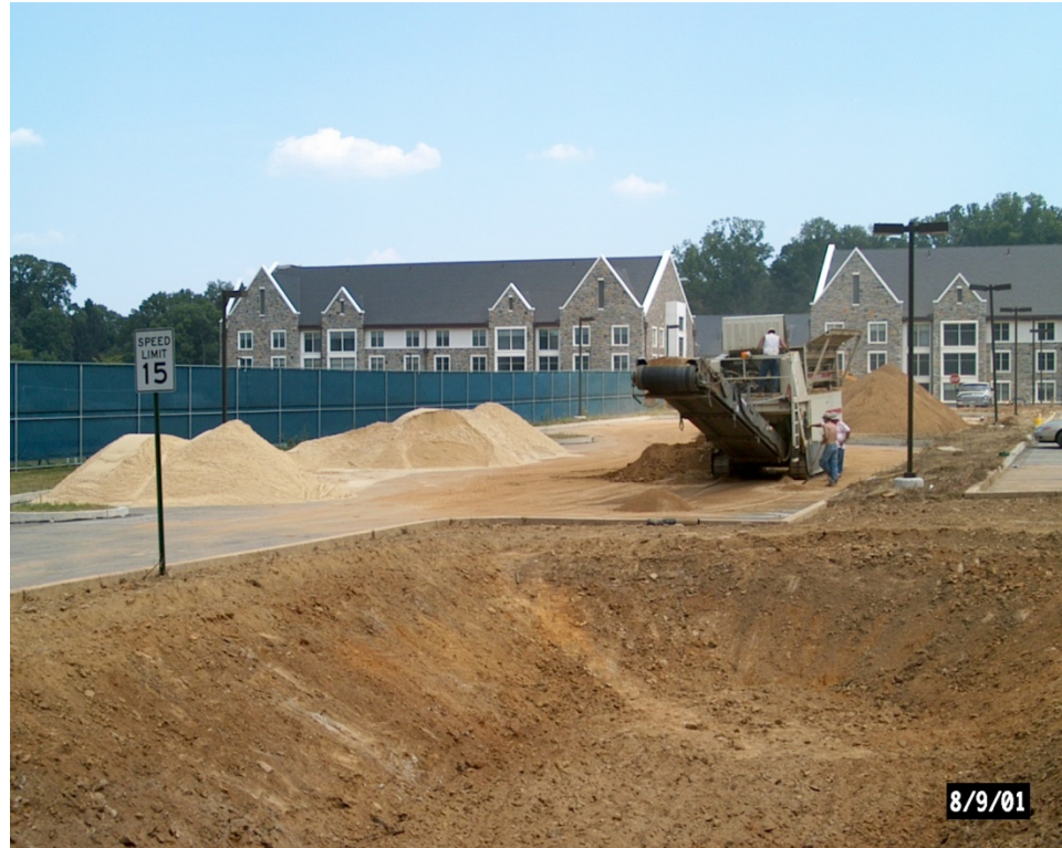
Figure 6. Excavated soil mixed with silica sand to create rain garden media
