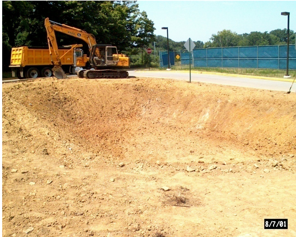
Figure 4. Excavation of traffic island to a depth of six feet
