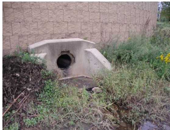
Figure 5.1: First inlet structure for Metroplex Shopping Center SCM
