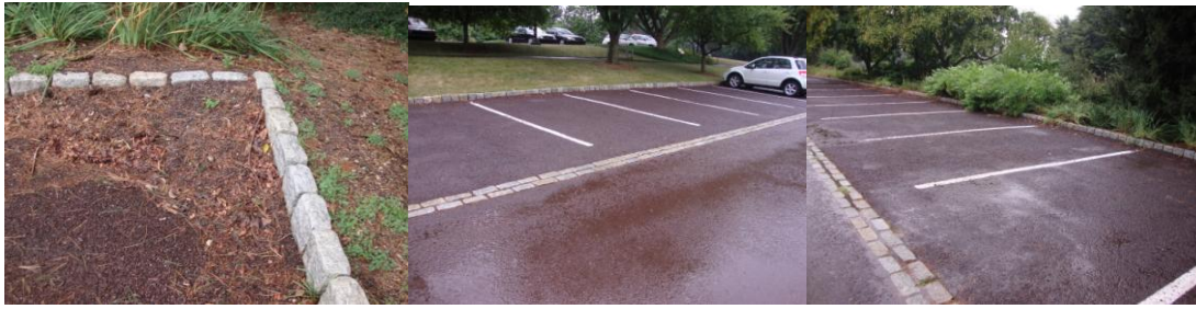
Figure 5.7: Sediment build-up and clogged areas at Morris Arboretum greatly affecting performance
