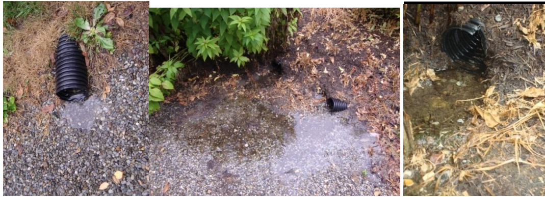
Figure 5.28: Inflow pipes routed from rooftop drain to seepage pit
