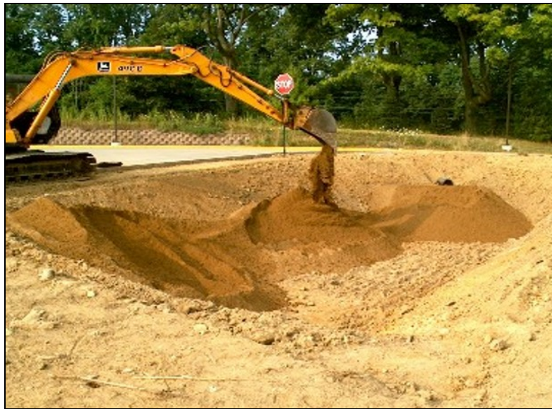
Figure 1-3: Addition of Mixed Soil during Construction
