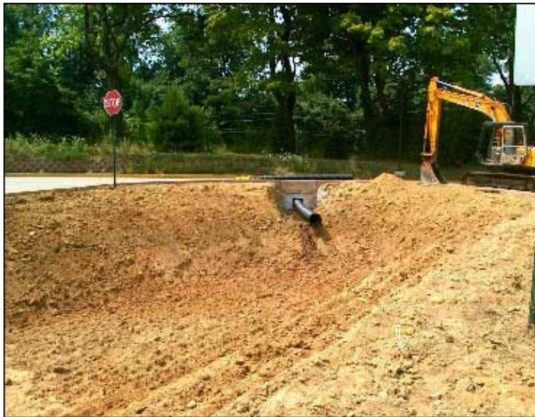
Figure 1-2: Excavation of Basin with Addition of 12” Pipe
