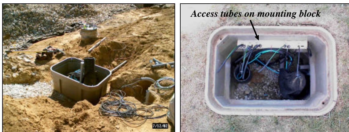
Figure 13. Access box during (left) and after construction (right)
