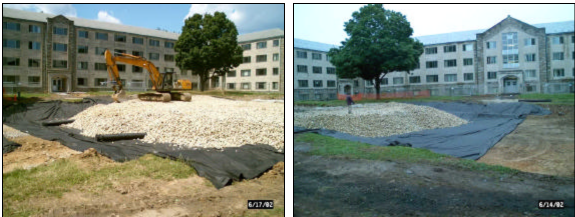
Figure 7. Photographs of infiltration beds during construction
