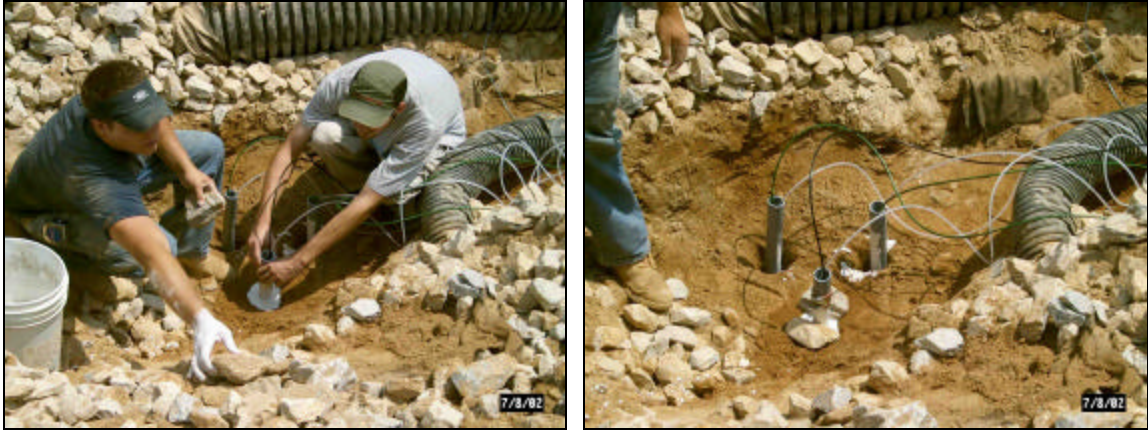
Figure 11. Installation of soil water samplers
