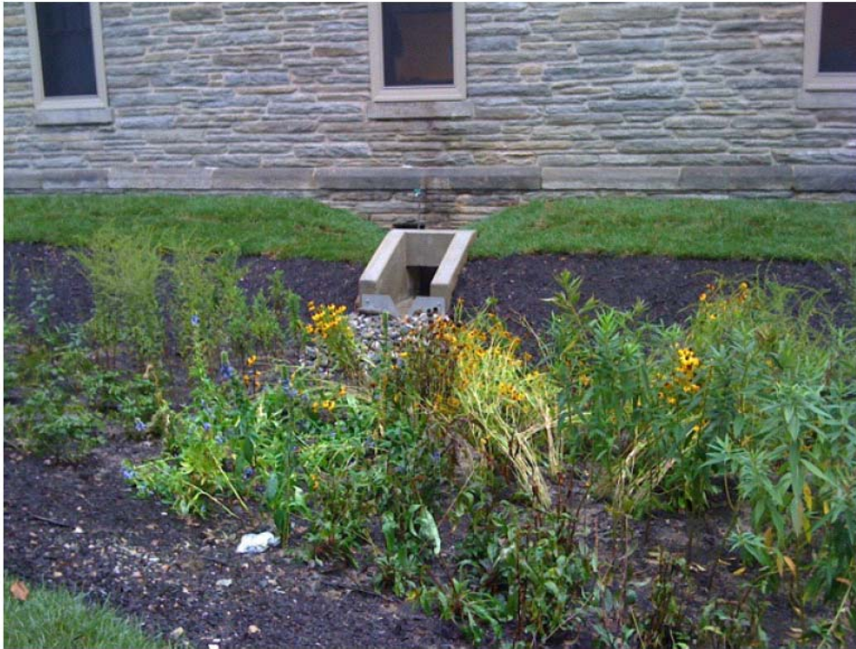
Figure 6.9 Fedigan bioinfiltration rain garden. Inflow V-notch weir shown.
