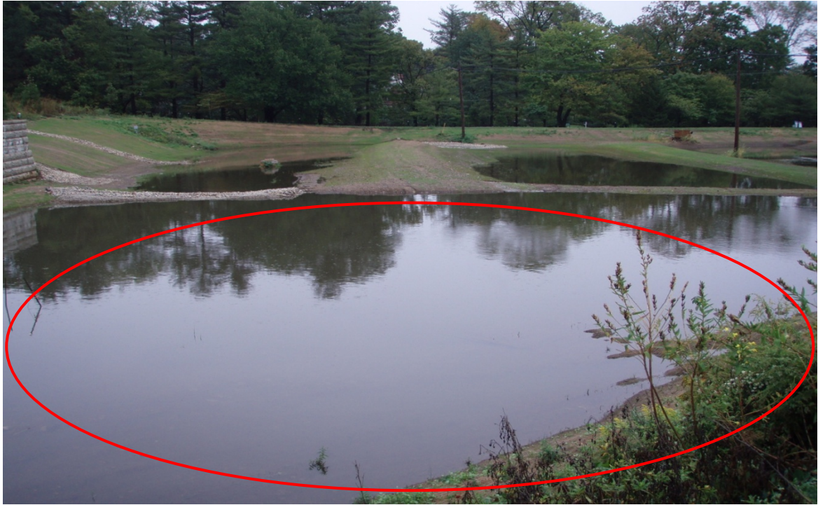
Figure 1-4 New sediment forebay with water at baseflow (circled in red). The first meander is to the left in the picture, and the second meander to the right.
