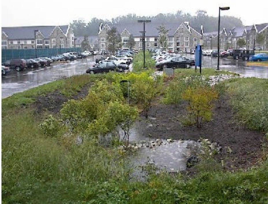
A9: Completed Traffic Island with vegetation and monitoring equipment.
