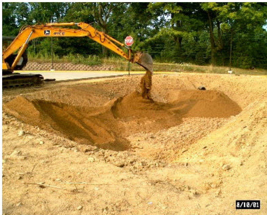
A6: Made soil is being added back into traffic island to form the infiltration bed.
