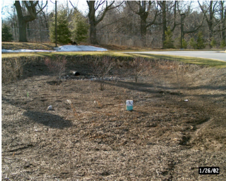
A13: 48 hrs later, all of the runoff has infiltrated.
