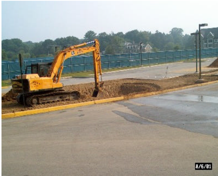
A1: Excavation of native soil. Curb cut placement is determined by flow of water across surface.
