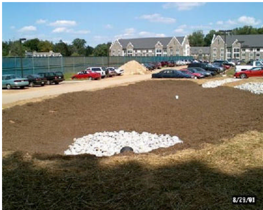
A8: Mulch is placed on top of the soil to prevent erosion until the vegetation grows in. Rip rap is placed along flow paths to further reduce erosion.
