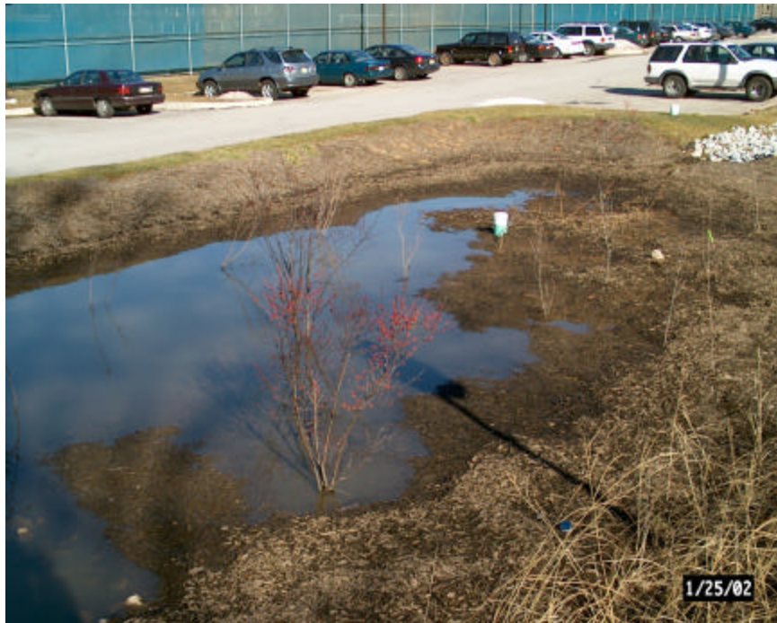
A12: Within 24 hrs, most of the runoff infiltrates.
