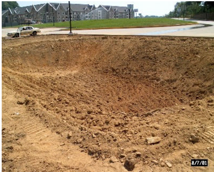
A2: Completion of excavation.
