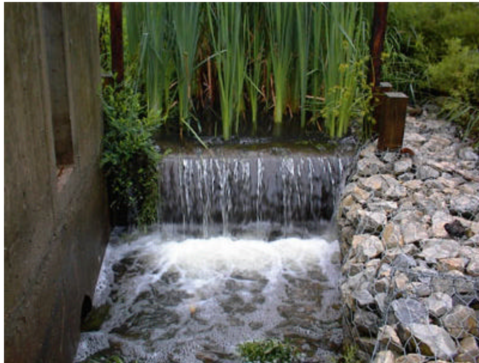
Figure 7. Modified outlet structure during moderate storm event
