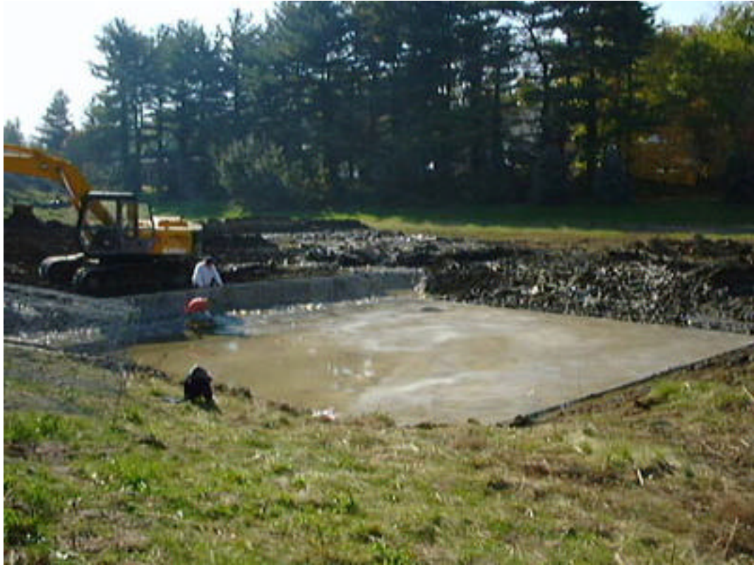
Figure 4. Concrete pad to form base of sediment forebay
