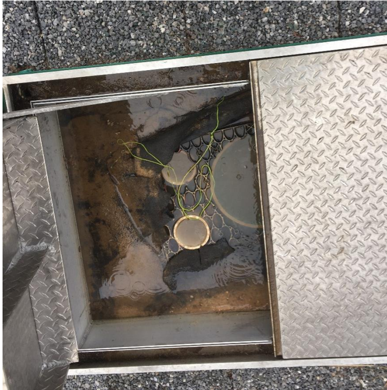
Figure 5.17: Treatment Train Infiltration Trench at Maximum Observed Level
