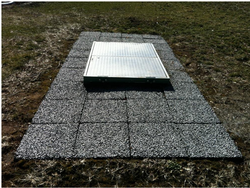
Figure 1.8: Treatment Train Infiltration Trench
