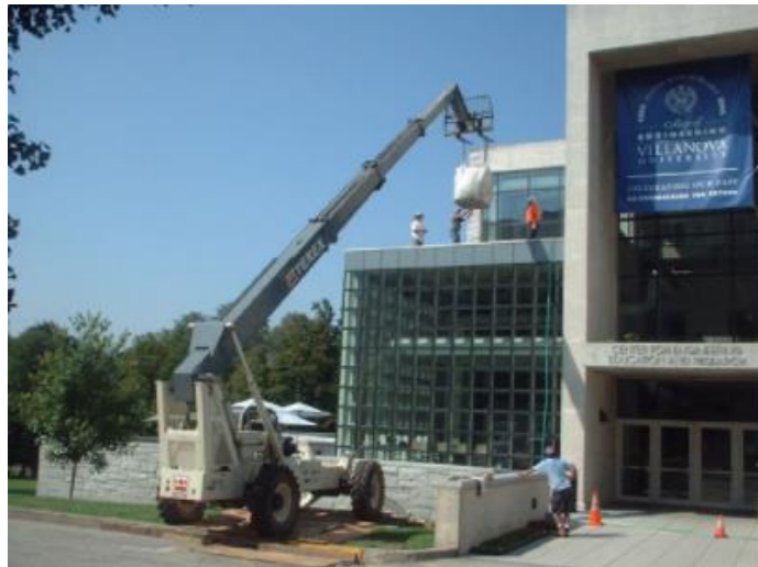
Figure 1.1: CEER Green Roof Construction
