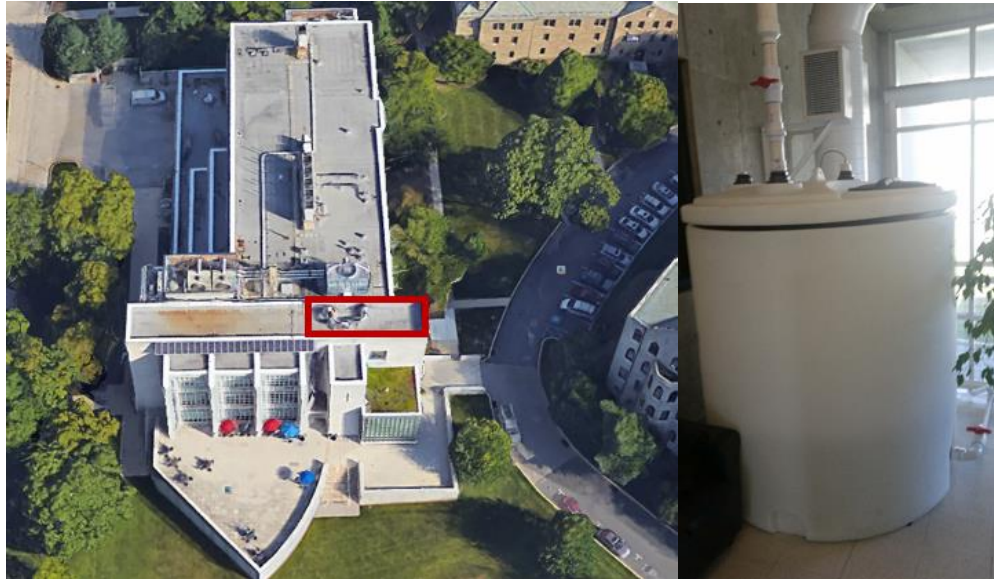
Figure 1.4: Drainage Area and Cistern Added to CEER Green Roof System with RTC Retrofit
