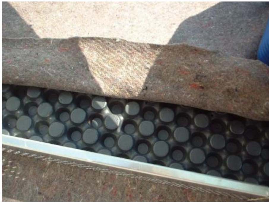
Figure 1.2: Geotextile and Drainage Layer of CEER Green Roof
