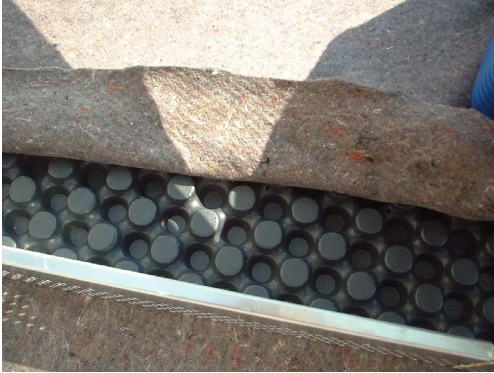
Figure 3.3: Optigreen Filter Fabric Overlaying Expanded Plastic Drainage Board (VUSP)
