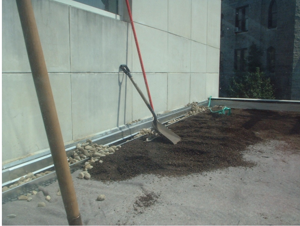
Figure 3.4: Installation of the Rock Perimeter Adjacent to Existing Wall. (VUSP)
